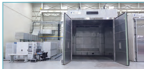
친환경선박용 추진체계 내환경 및 안전성 시험평가 설비 Facility for testing the anti-environment and safety performance of the propulsion system for eco-friendly ships
